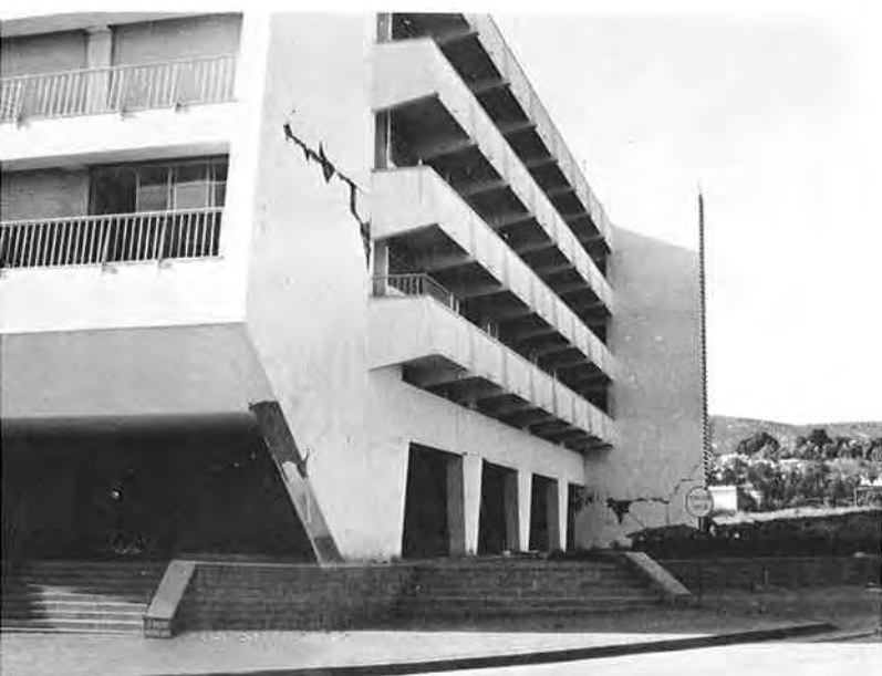
Fig. 62. Immeuble Paternelle, from the Southeast
