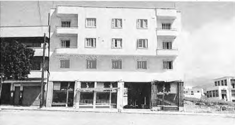
Fig. 68. Racking of Reinforced Concrete Columns
