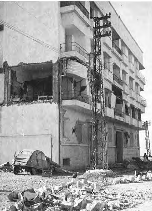
Fig. 70. Reinforced Concrete Frame Carries Load in Spite of Damage to Masonry
