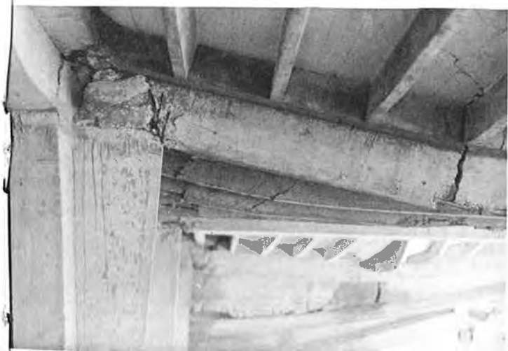
Fig. 67. Detail Demonstrating Large Yield Capacity of Market Frame Structure
