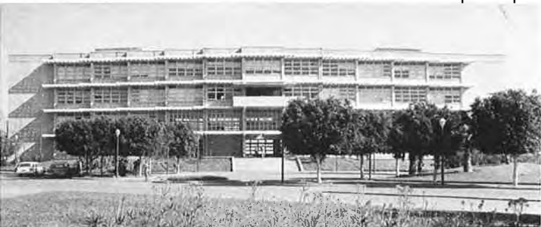
Fig. 52. Agadir Municipal Building, After the Earthquake
