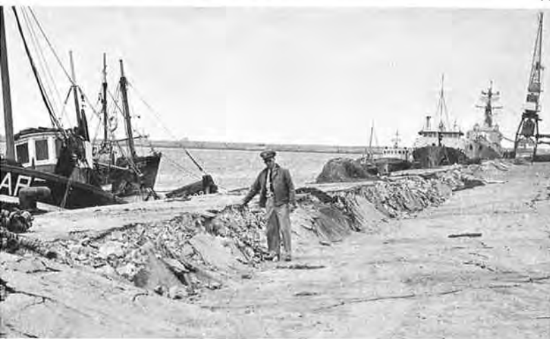
Fig. 83. Subsidence of Fill Adjacent to North Quay Wall
