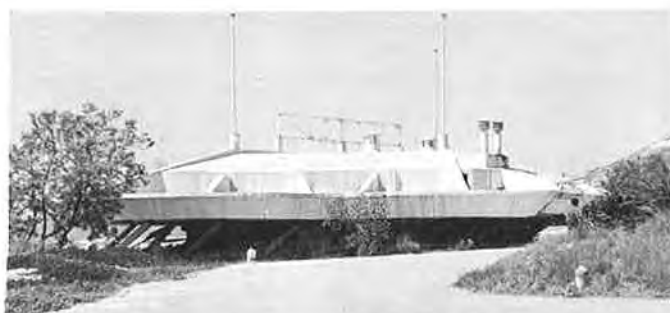
Fig. 73. "La Reserve" Restaurant From the East, After the Quake
