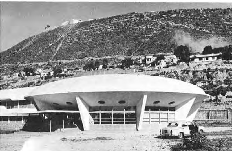
Fig. 76. The Customs House in the Port Area, After the Earthquake
