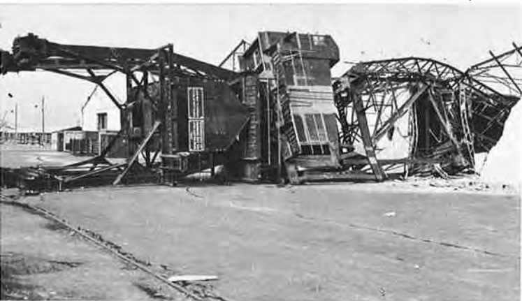
Fig. 89. Warehouse Building Crushed by Overturning of Crane
