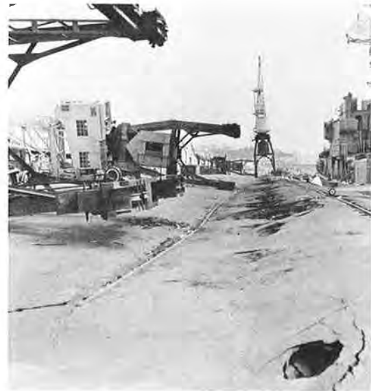
Fig. 87. Tilting of Crane, North Quay Wall
