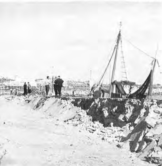
Fig. 82. Subsidence of Fill Adjacent to North Quay Wall
