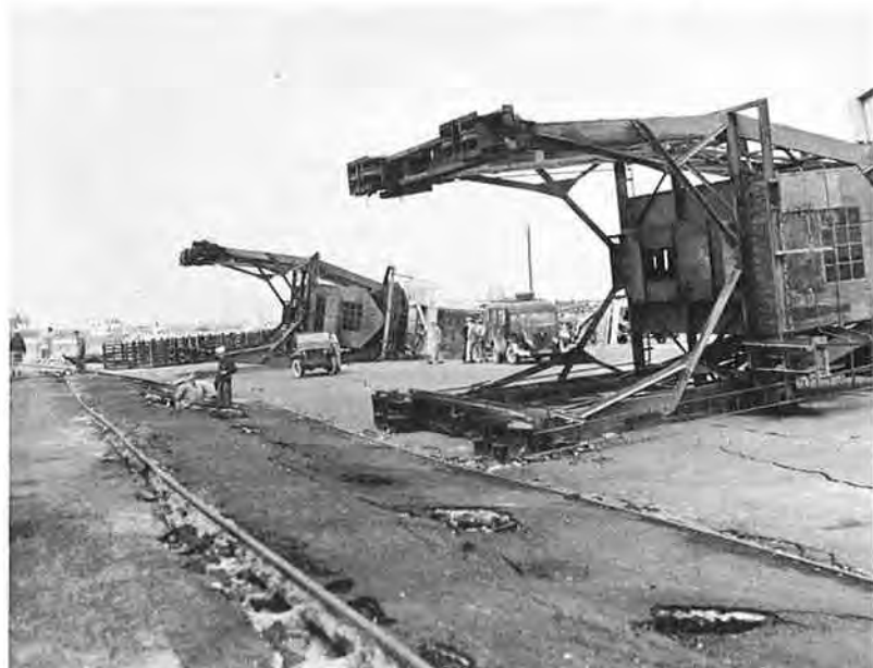
Fig. 86. Cranes Overturned by Fill Subsidence, North Quay Wall
